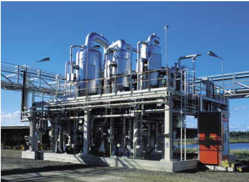
A three-effect system that evaporates NaOH from 32 to 50% at Akzo Nobel in Sweden. The system was built by the contractor Chematur Ecoplanning, using AlfaVap and AlfaCond. The need for exotic materials such as nickel makes the AlfaVap exceptionally economical in this application.
